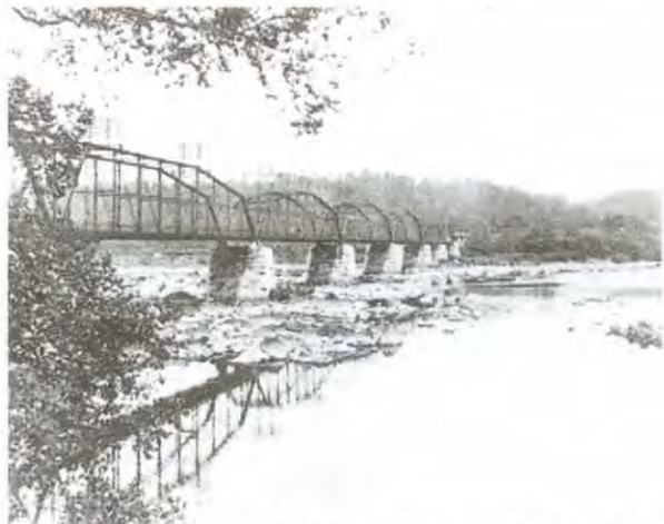
The Old Truss Bridge at Conowingo (courtesy of the Harford Historical Society).
